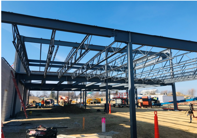
Setting Steel Beams & Joist, Administration Area
