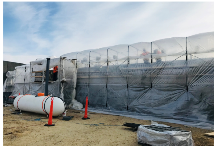
Masonry Enclosure for Laying Interior Masonry Block, Kitchen Area
