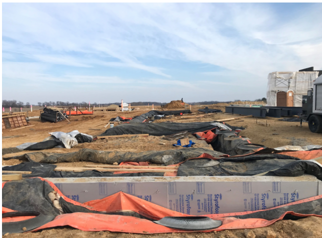
Forming & Pouring Foundation Footings, Commons Area
