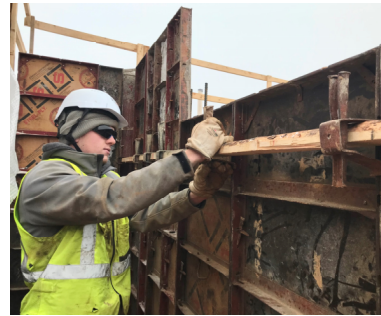
Tony Wolf , Assembling Symons Steel Ply Forms Ahead of Pouring Concrete for the Loading Dock Foundation Wall.
